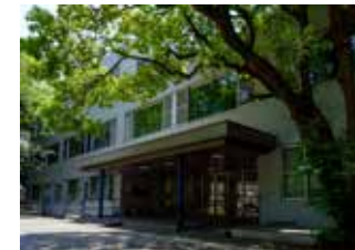
美術学部中央棟 Main Building, Faculty of Fine Arts
